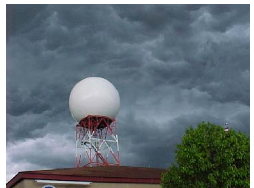
The WSR-88D radar at the NWS Forecast Office in Romeoville.
