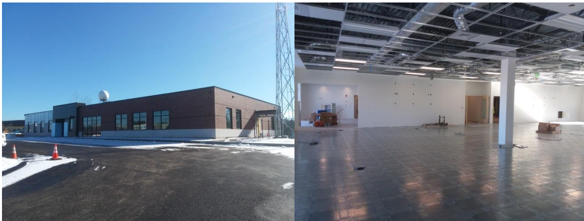
New NWS facility under construction in Norton, MA
